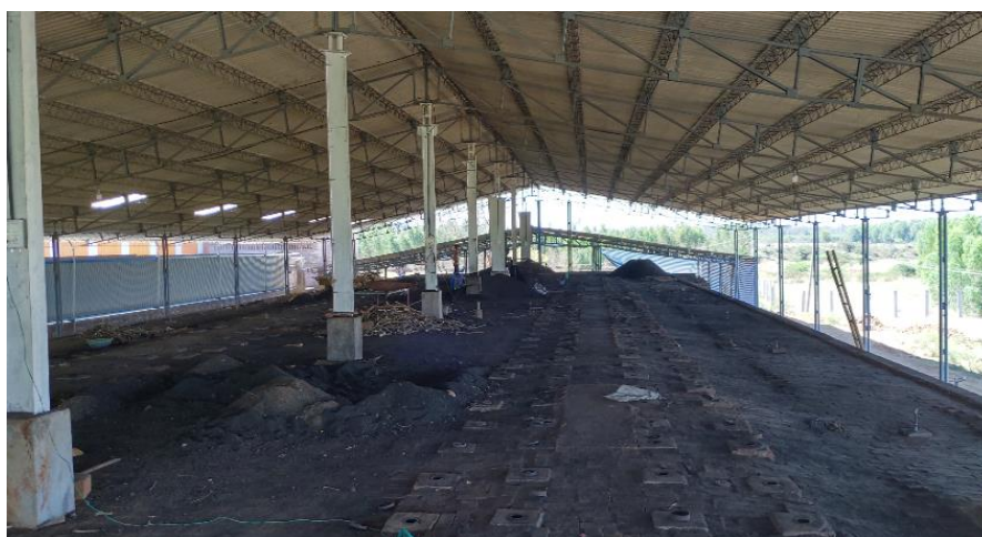
FIGURE 40 HHK AT FORTE BRICKS
