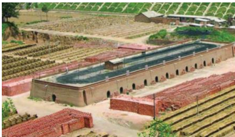
FIGURE 19 PICTURE OF HYBRID HOFFMANN KILN (HHK)
