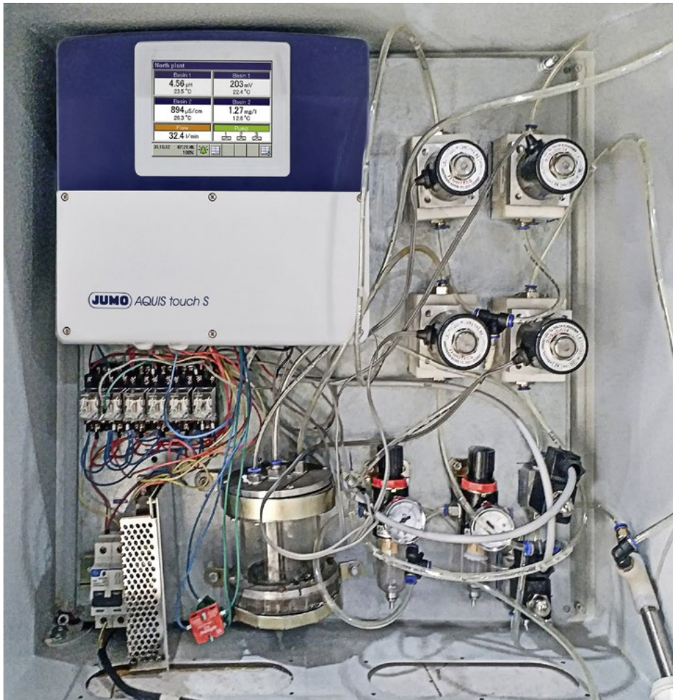
Figure 2: JUMO AQUIS touch S modular multichannel meter with integrated controller and screen recorder
