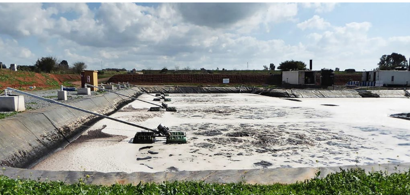
Figure 1: Conversion to OxyStar aerators at the Oum Azza leachate treatment plant, Morocco
