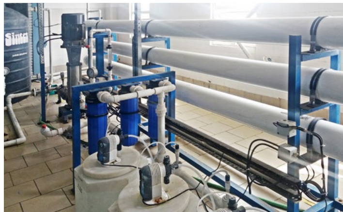
Figure 1: Structure of membrane stage using ZLD technology in plastic electroplating (left) Photograph of RO stage 1 (right)
